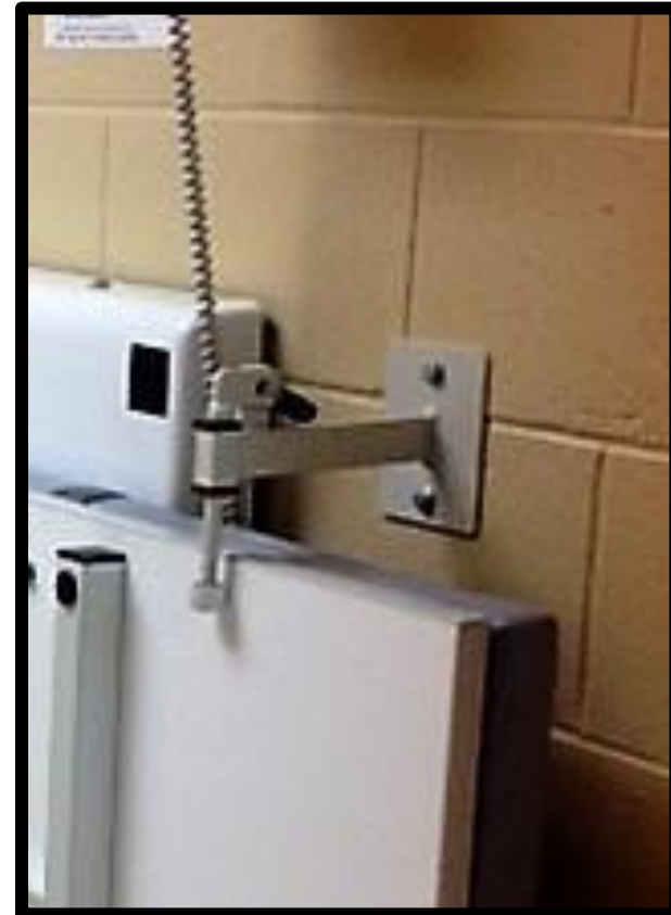
Close-up of Safety Locking Bracket
